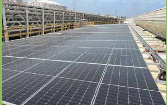
▲ Newly solar generation facilities on the roof of plants in the Mailiao plant site
