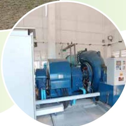
▲ Newly hydropower generation facilities on the roof of plants at Shalu Water Supply Center (Power generator)
